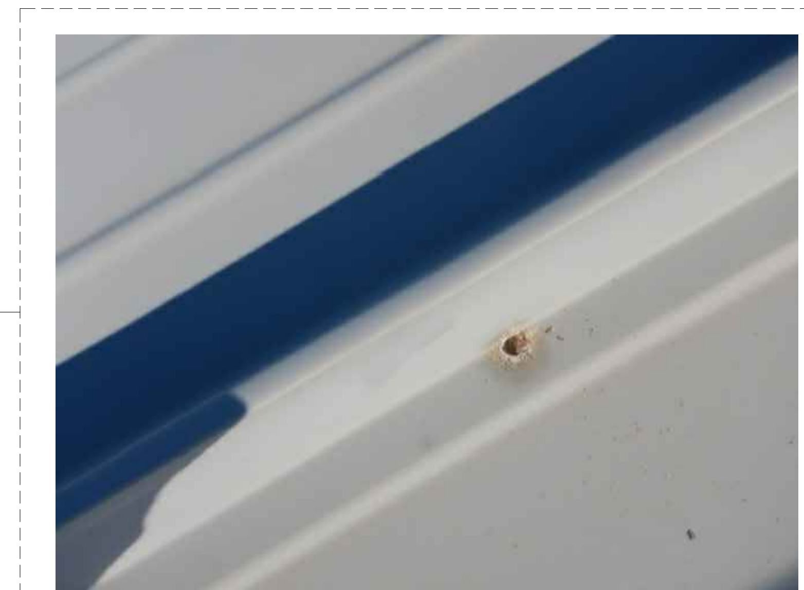
E PHOTOGRAPH OF TYPICAL DAMAGED COATING LOCATION SCALE: NTS
